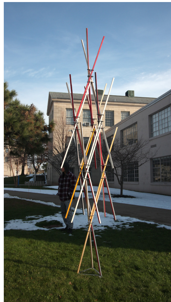
Full scale mock-up (8 blocks complete 1 rhombohedral structural module. 12ft, 3.7m tall)
